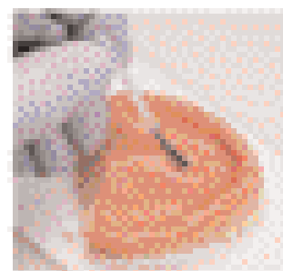
1. Coat Maxcush Bonding Liner
