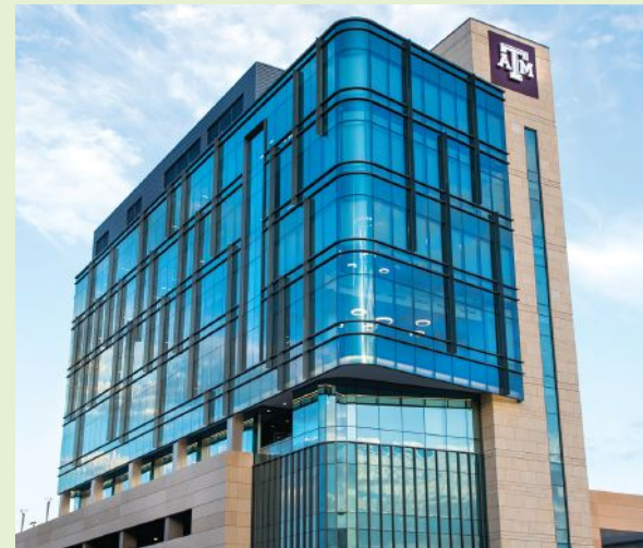
First: The Clinic and Education Building, which features nearly 300 dental chair stations, is the first stand-alone building constructed for the dental school since 1950.
