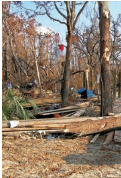
Moving on: All that remains of Dr. Drake's home in Pass Christian, Miss., are some posts.
